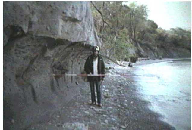
Figure 5: Formation of a concave erosion zone due to wave erosion, and the resulting overhang at Site 1.
