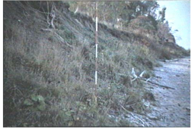
Figure 8: Stable slope at Site 2 due to colonization with grasses and shrubs, thereby reducing sub-aerial erosion.
