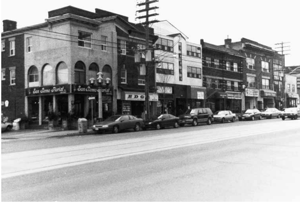
Figure 5. A typical block face on St Clair Avenue, displaying a hybrid mix of Georgian and Italian-Canadian architectural features. Author's photograph, autumn 1996.
