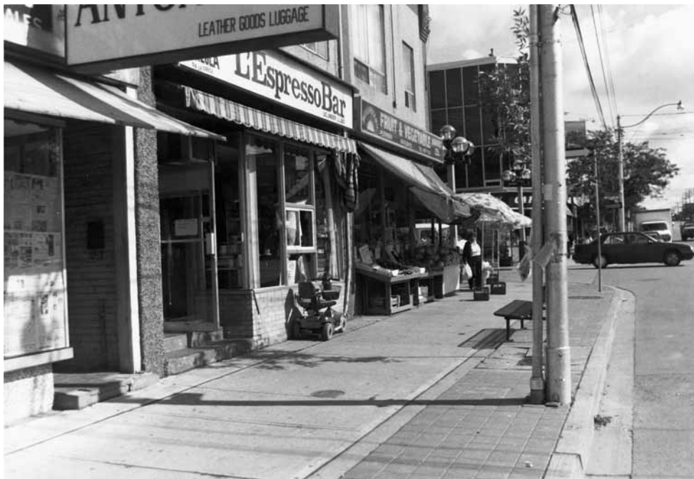
Figure 4. Removal of central vestibule and the installation of a plate-glass window with a café window. Author's photograph, autumn 1996.
